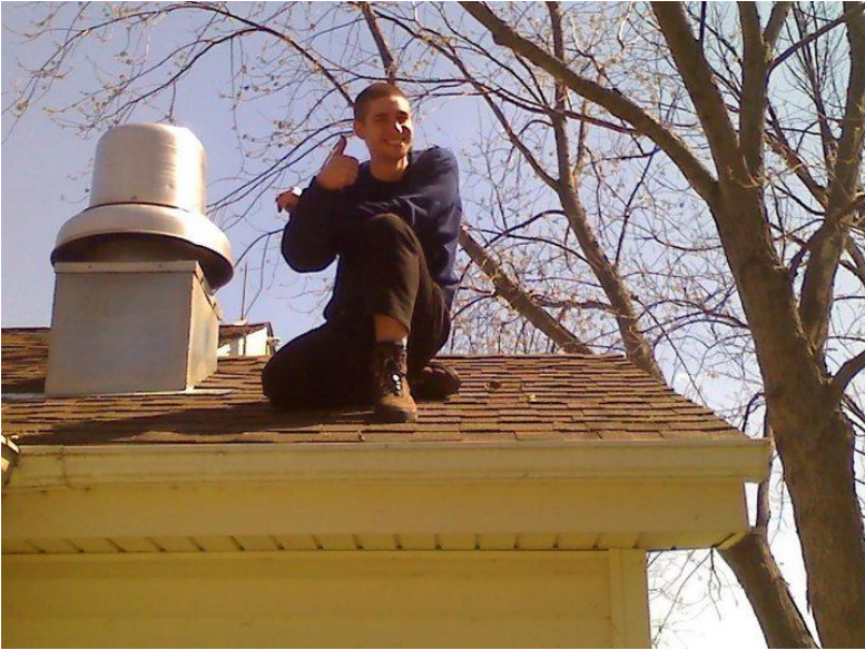
A thumbs-up while clearing the rain gutters of the dining hall.
